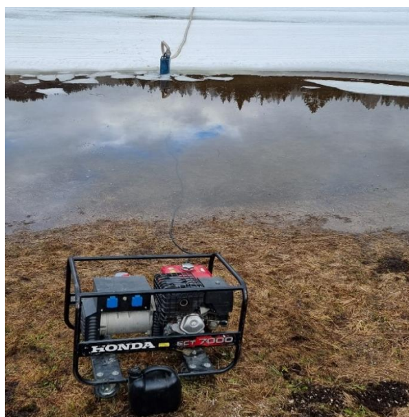
You know you're in trouble when they start pumping water off the track!
